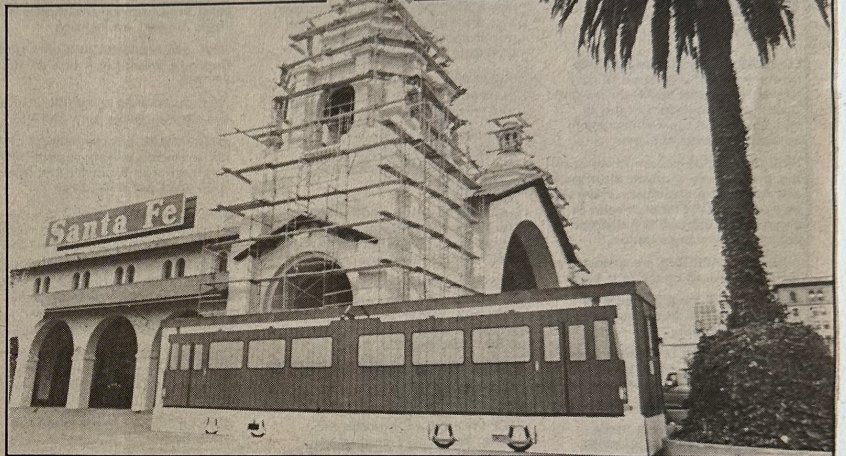
OTHER PROJECT /Art Cole has created yet another trolley mural. This on the construction shed at the Santa Fe Depot.
